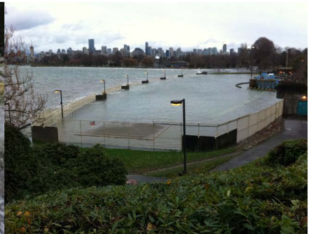
Inundation at Kitsilano Pool, City of Vancouver
